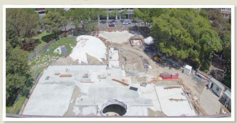
View from top of the Anzac Memorial towards Liverpool Street showing completion of the precast structure and formation of the new oculus and cascade walkway.
